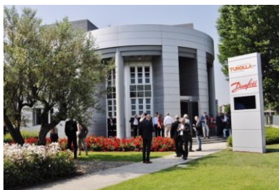
Picture from the Grand Opening of Turolla's new facility – the main entrance.
